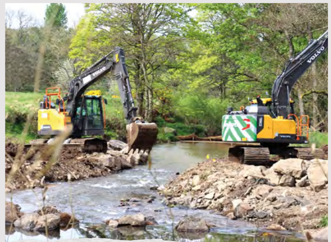
ABOVE: Diggers removing the Burn of King Edward weir
