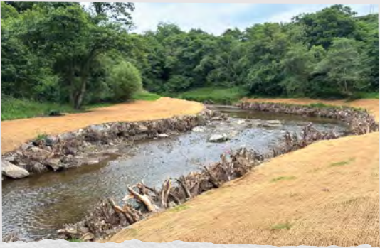
ABOVE: The riverbanks were stabilised with boulders and locally-sourced wind-blown trees.
