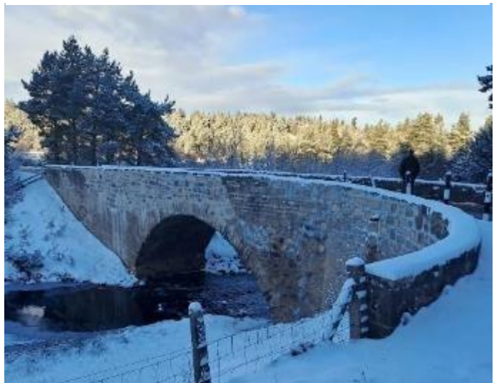
A939 bridge at Dava station fully repaired, Jan 2024. (photo Sean Mclean)
