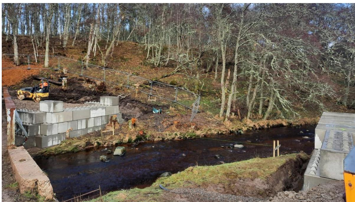
*Photo 2: Supports for the new bridge at Inverbrough constructed from [EuropeBlocks](#), Jan 2023. (photo Sean McLean)*
