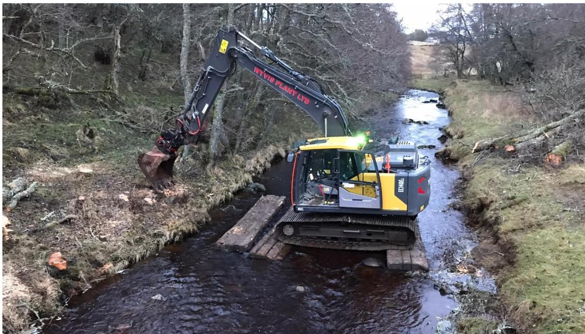
*Photo 2: Novel technique used by contractors to minimise bed disturbance on the Allt Bruachaig, during construction of the new bridge at Inverbrough, Jan 2023. (photo Sean McLean)*
