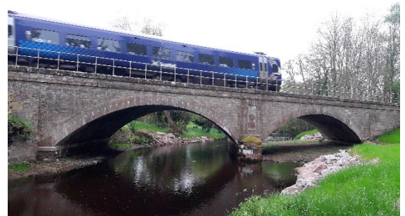
Bridge repairs completed.
