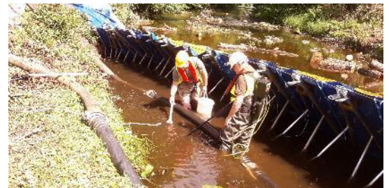
Prior the site being pumped dry a fish rescue is carried out using electrofishing. All fish captured are released to a nearby area outwith the works area.
