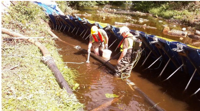
Fish rescue underway at the Brodie Rail Bridge June 2022.
