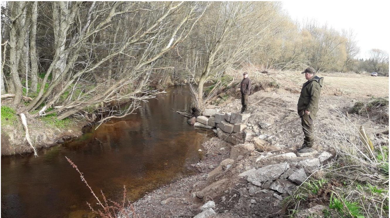
Sean and Ali inspecting river works at Banarach Bridge on the lower Muckle Burn, where waste concrete was used to provide bank protection and the channel deepened.
