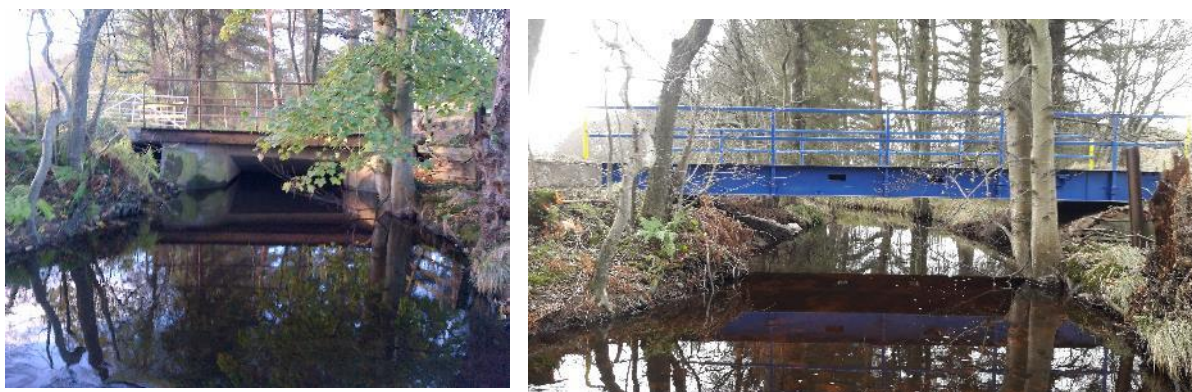
New bridge at Burnside Cottage on the Black Burn improves fish passage and reduces localised flooding. Old bridge on the left, new bridge on the right.
