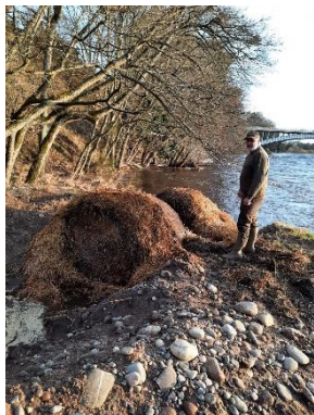
Straw bales used to control siltation during drain clearance on Dalvey Estate.
