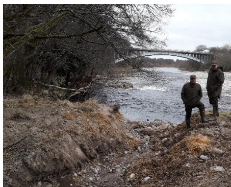
Straw bales used to control siltation during drain clearance on Dalvey Estate.
