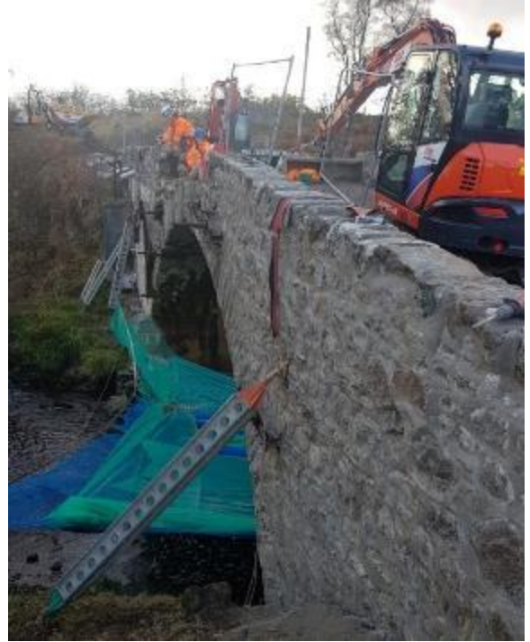
Repair works underway at Bantrack Bridge, Oct 2020. (photo Sean Maclean)
