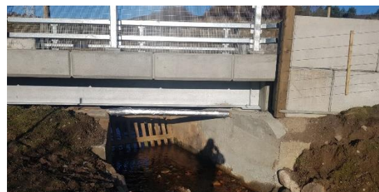
New bridge over Corrievorrie Burn. (Photo Sean Maclean)
