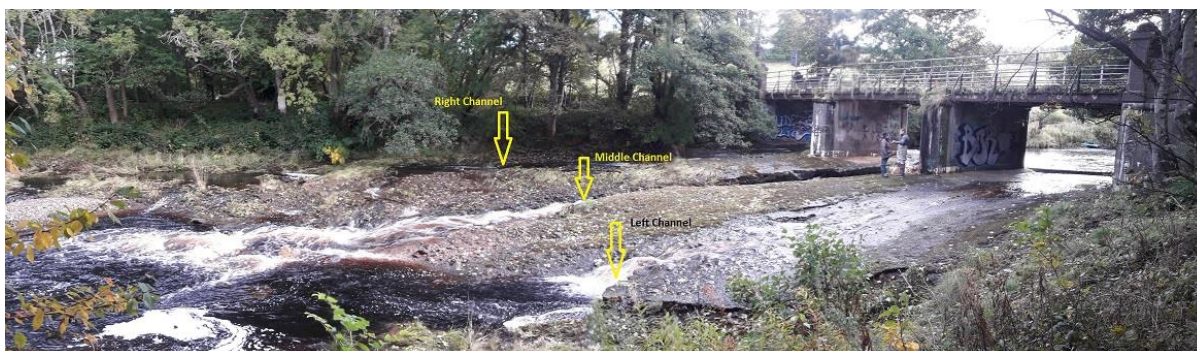
Photo 2: Cloddach Bridge medium flows 2020-10-09
