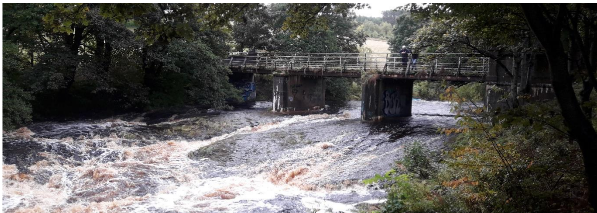
Photo 1: High flow at Cloddach bridge 2020-10-05
