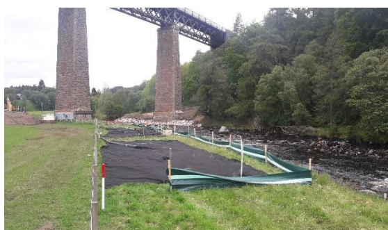
Large geotextile bags used for silt control.
