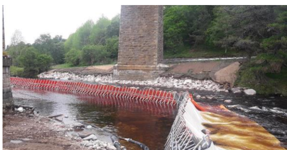
Portadam installed around left bank pillar June 2020.
