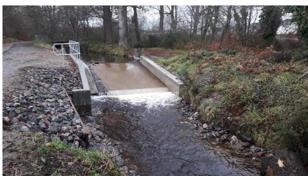
New weir and fish pass at Linkwood Distillery.
