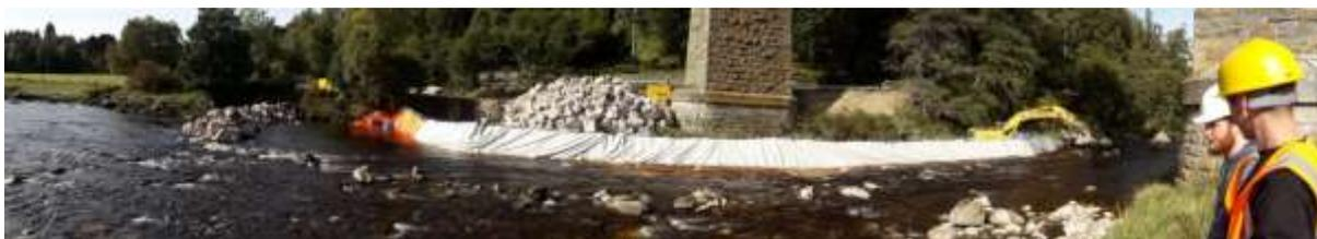
*Installing the portadam around the right bank pillar of the Tomatin railway bridge, Sept 2019*
